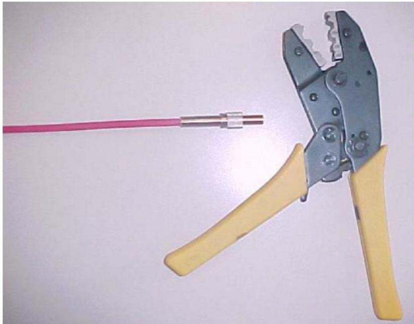
Press with the pliers the metal cover connector on the ring
